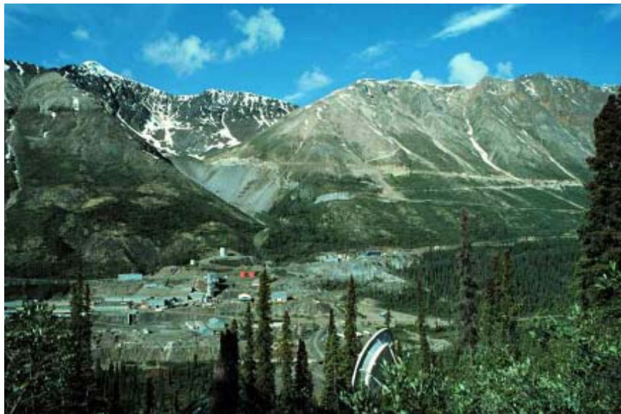
Figure 2.5 Cantung Mine near Nahanni
